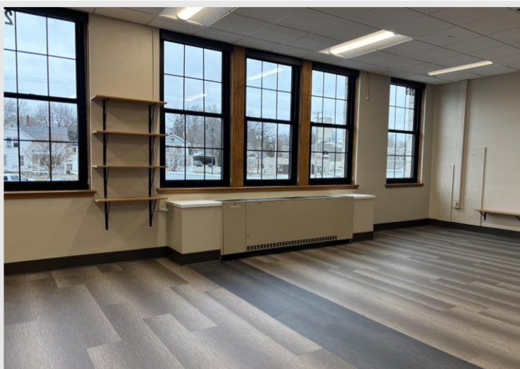
New unit ventilator installed with wingwall countertops on top of the new flooring system!
